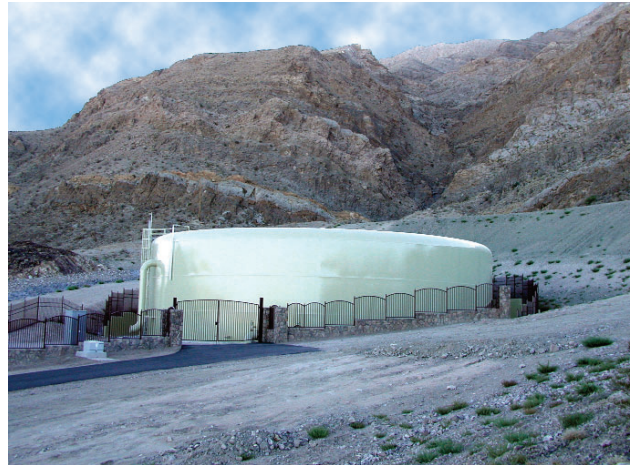
Baro Canyon Reservoir
