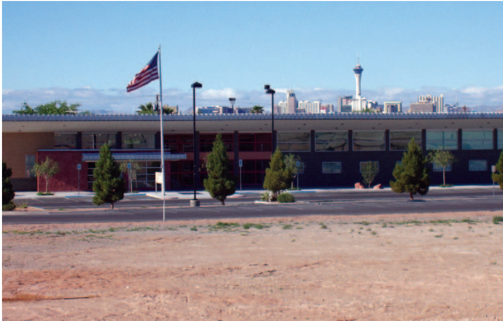
Sumter Utility Building
