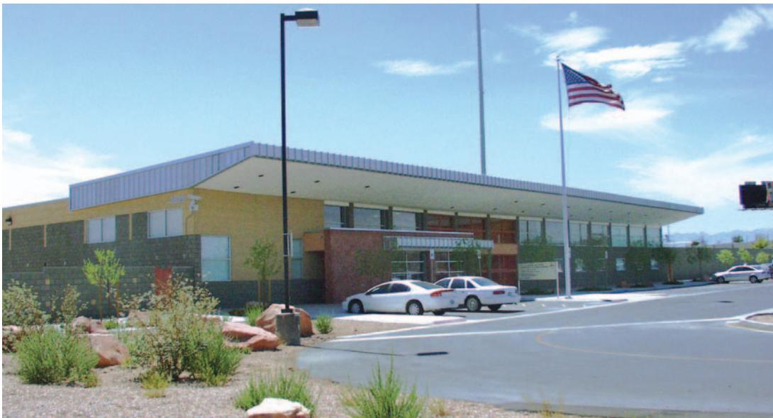
Fort Sumter Utility Building
